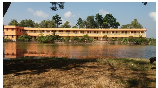
Mission has constructed an oldage home for the helpless old people.
